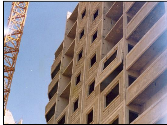
Photo 4. Carrying the precast panel wall to its place [Archive of Korur]
