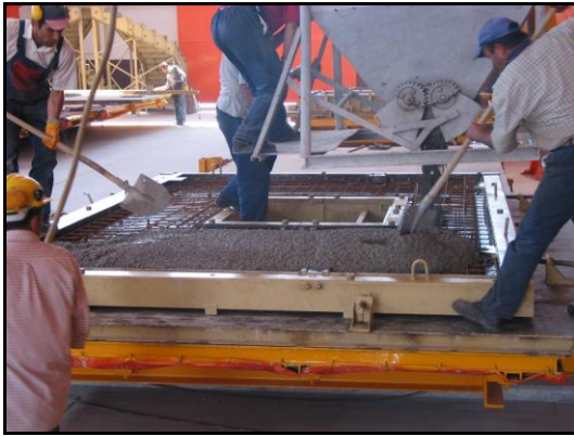
Photo 3. Production of precast panel wall on vibratory table [Archive of Korur]
