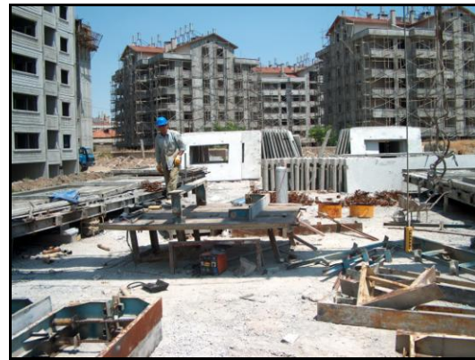
Photo 2. Casting precast element atelier established in-situ [Archive of Korur]
