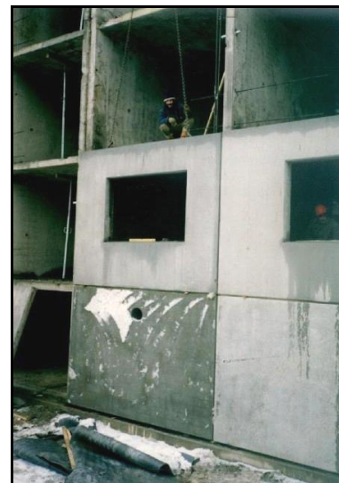
Photo 6. Application of Sandwich panel walls [Archive of Korur]
