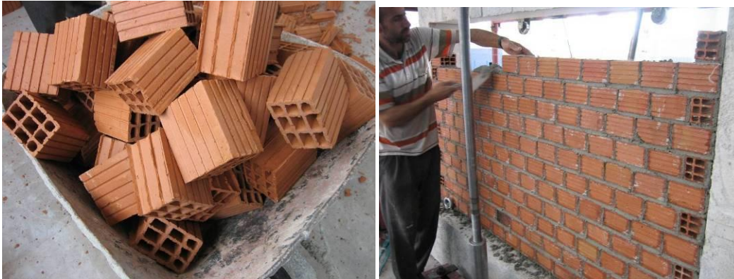
Figure (6) 1/2 scaled bricks were used with ordinary mortar
