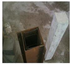
Fig.2 Concrete jacket before casting
