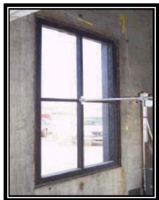
Fig. (8): Interior view of a Muntin window during test.
