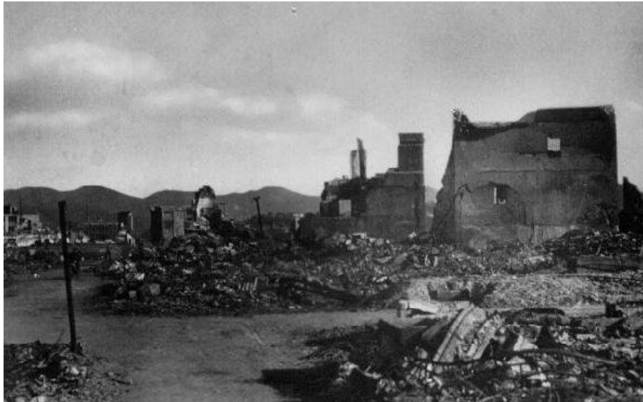
Fig. (1) The damage in Nagasaki after the nuclear explosions
