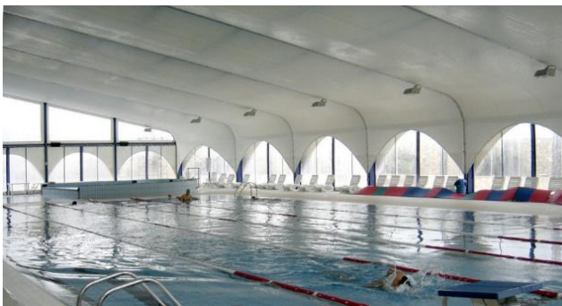
Figure 3: internal portal frames
