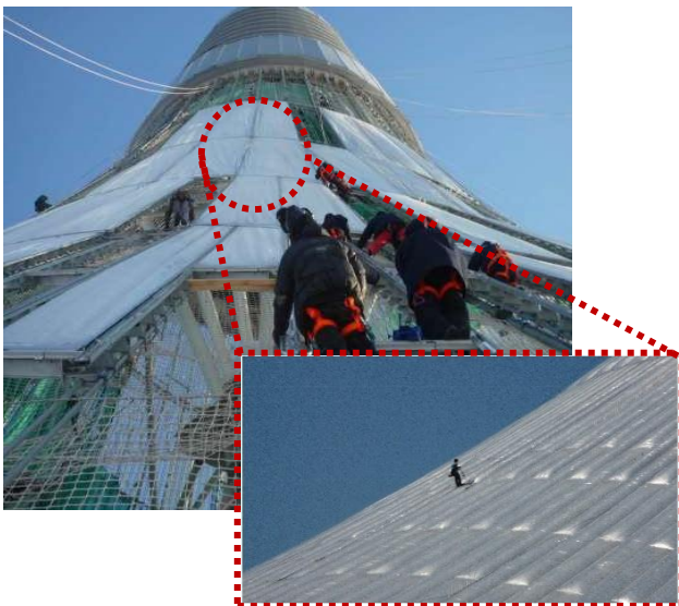
Figure 27: Material Construction. Source: fosterandpartners.com
