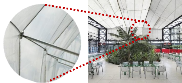
Figure 11: Research Center Coating Material.
