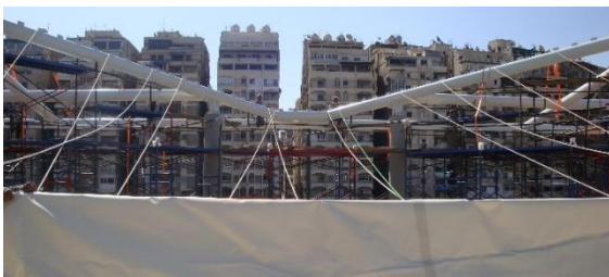
Figure 7: Specific Technology to install the roof of Sidi gaber terminal
