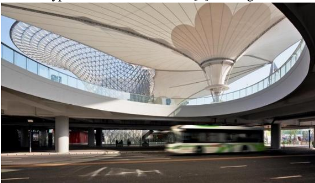
Figure 23: Natural lighting at the central spaces. Source: archdaily.com (Adapted by researchers).
