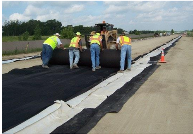
Fig (2): Geo-textile in road construction (19)
