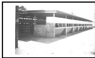
Diagram (1): Semi-open barn Diagram (2): Front Layout of the semi-open barn (1) Asbestos roof. (2) Ventilation opening. (3) A short wall. (4) Concrete floor.
