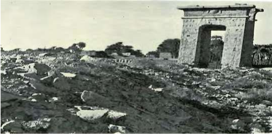
Fig (1): The temple before the excavations
