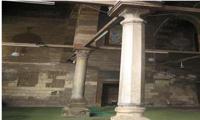
Figure (10) An example of a Corinthian capital from the interior of al-Maridānī mosque
