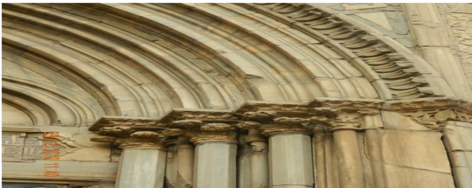
Figure (2) The multi layer retrograde pointed arch of the Gothic portal along with the Gothic style capitals
