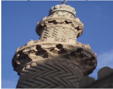
Figure (9) The deep zigzag motif of the west minaret
