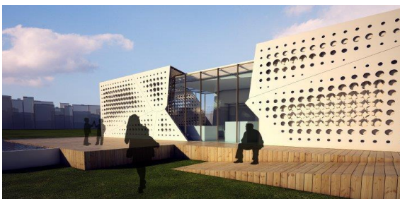
Fig. 1: Exterior of the base-case (slides house).
