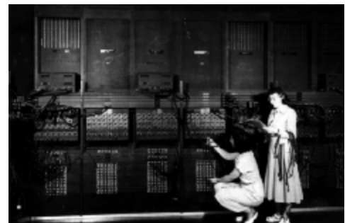
Figure 05 beginning of computer manufacturing the Electrical Numerical Integrator and Computer completed in 1945. source ( www.dreamhost.com )
