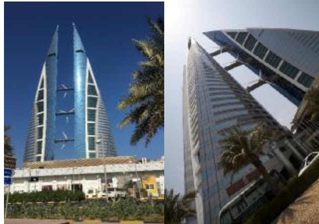
Figure 15 Bahrain WTC the first skyscraper in the world to integrate wind turbines into its design. Source ( http://www.designbuild-network.com )
