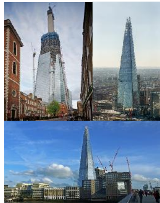
Figure 18 The Shard London Bridge designed by Renzo Piano and engineered by Arup and WSP Canto. Source ( www.designbuild-network.com )
