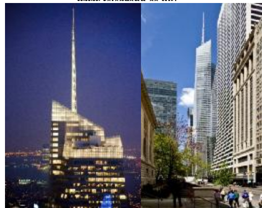
Figure 13 Bank of America tower . Source ( http://www.skyscrapercenter.com )
