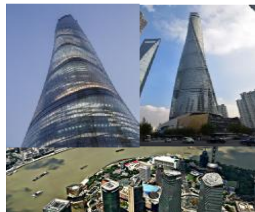
Figure 14 the tower's swiveling, asymmetrical glass façade confuses the organization of wind forces. Source ( http://www.skyscrapercenter.com )
