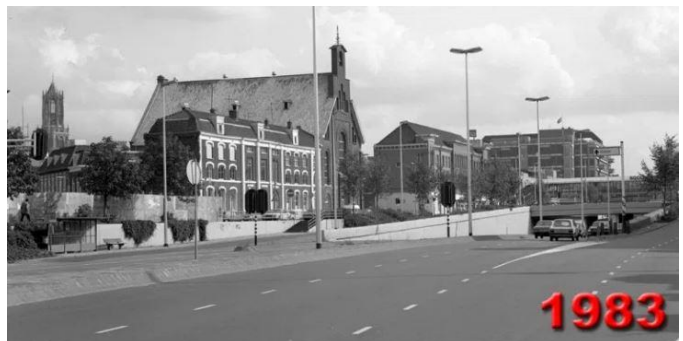
Fig. 18: Utrecht's motorway which located above the dammed canal [13]:
