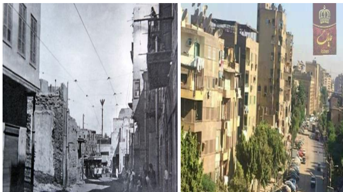
Fig. 29: Port Said Street after filling al-Khalij al-Masri canal [20] and [21].
