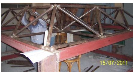
Figure 4: Assembling process of truss#1 members
