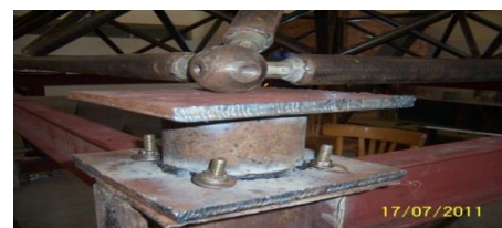
Figure 5: Connection between truss#1 and supporting frame
