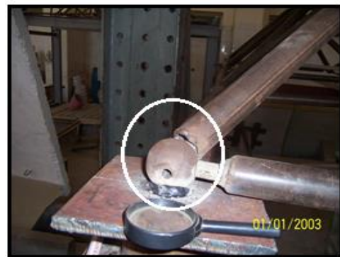
Figure 19: Collapse in the corner member from the first test of truss#1
