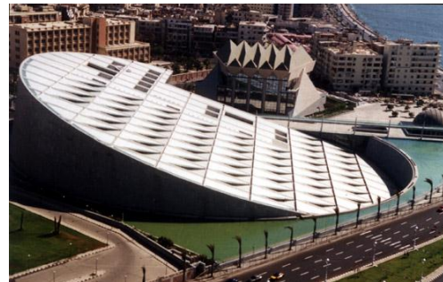
Fig (6) The inclined roof which forms a challenge for maintenance processes Source: Researcher
