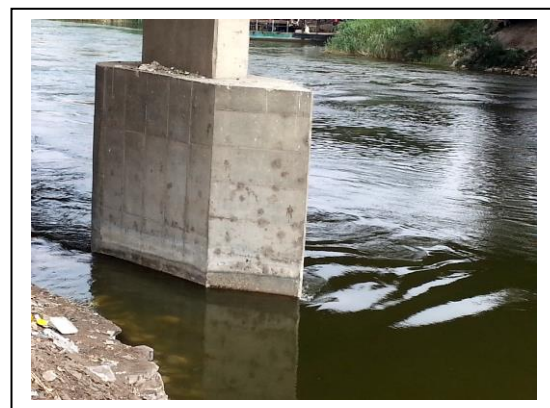
Photo (2) Mataria bridge at Cairo-Egypt
