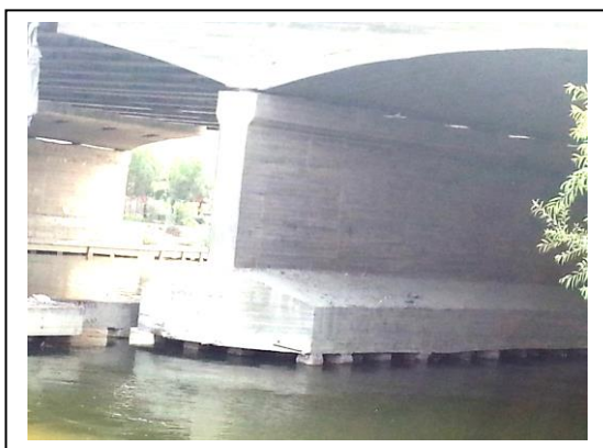
Photo (1): Mestored bridge at Cairo-Egypt
