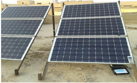
Figure 11: Installation of PV array
