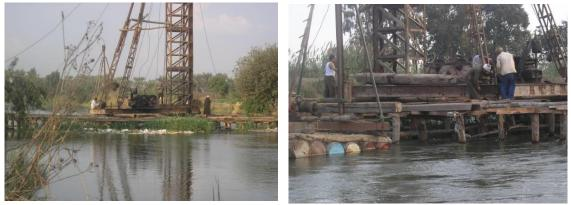
Fig. 11 Platform setup used to drive piles of bridges across water courses
