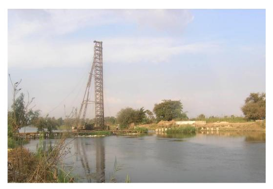
Fig. 3 Driven piles of the bridge in the North East of Egypt
