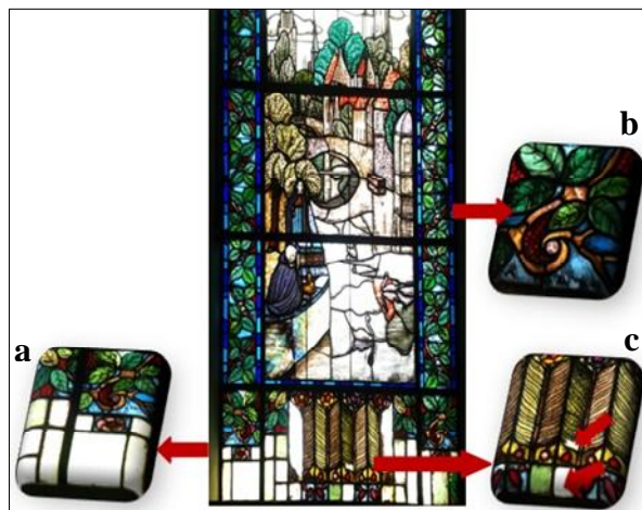
Fig. (4) Shows a . colored glass pieces were replaced with transparent ones, b . dust and dirt behind the panel causing darkening, c . clearest degradation manifestations is the loss of the green color under the panel.
