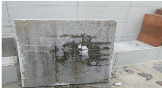
Figure(15-a): The crack pattern for slabs S3
