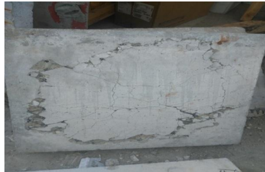
Figure (13): Shape of failure for slab S 22
