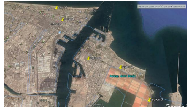
Figure 21: Working areas in Port Said
