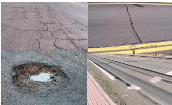
Figure 1: samples of road distresses
