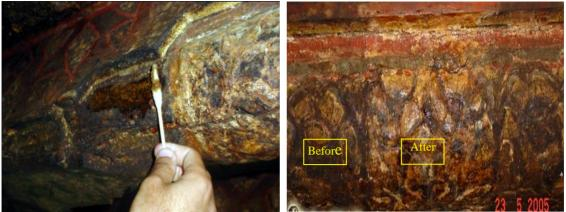
Figure (18) the chemical cleaning of the painted ceiling. 5.3.2. Sterilization
