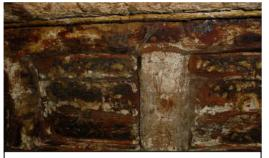
Figure (3) the formation of detachments and cracks of the wood ceiling due to temperature and humidity changes.
