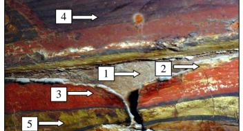
Figure (2) separation of all layers from the ceiling wooden support of Qaitbay's madrassa and shows multilayer system of the painting at the ceiling. <u>1</u> wooden support, <u>2</u> preparation layer, <u>3</u> red pigment, <u>4</u> yellow pigment, <u>5</u>blue pigment, <u>6</u>the gilded parts.
