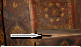
Figure (7) the warps, twists and shape distortions of the ceiling.
