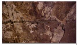
Figure (8) loss of some architectural elements as a result of biological attack at the ceiling  $\underline{a}$  bat droppings  $\underline{b}$  extracts of birds  $\underline{c}$  Bees nests
