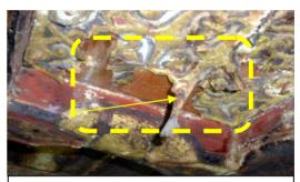
Figure (4) separation of painting layer of the ceiling.
