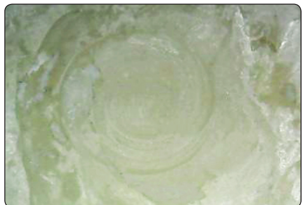
Fig. (4) Adhesive failure
