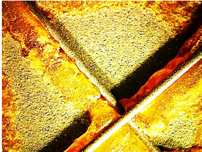
Fig. 14 Accumulation of polyurethane to the side of steel wire.
