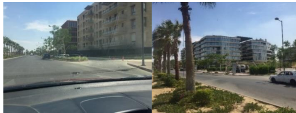
Figure (13) Beverly Hills. Services roads and parking shades
