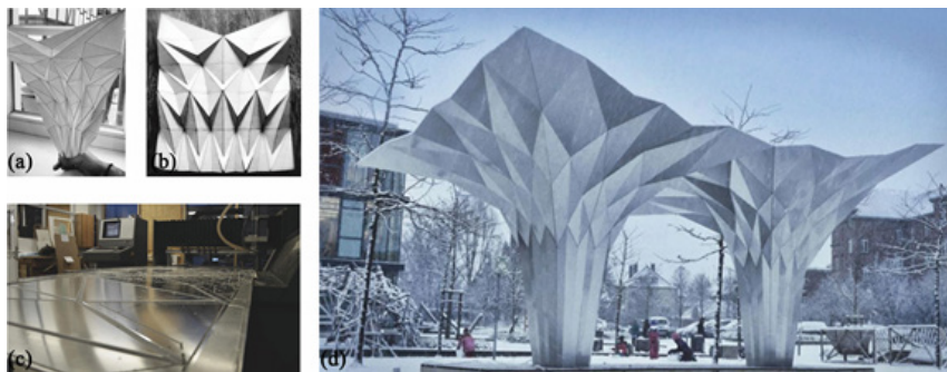
Figure 9: (a) (b) Prototypes of the principle in paper and cardboard, (c) CNC-milling the folding pattern into ACM boards, (d) Origami pavilion on the Campus Emilie in Detmold (16 pp. 177-183).
