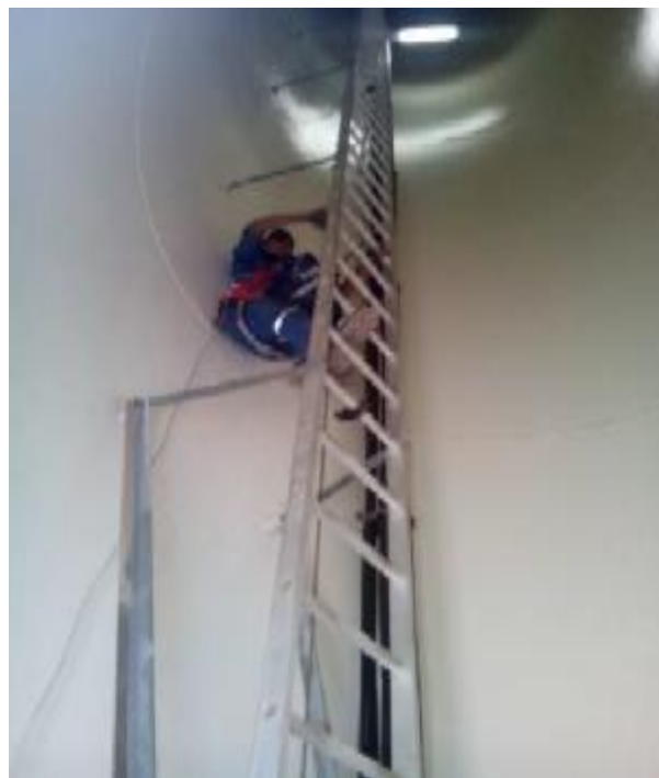
Figure (10) Working accessible space inside the tower
