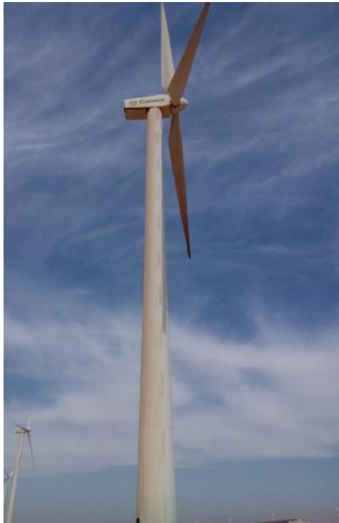
Figure (5) Gamesa G52 wind turbine towers at Zafarana (6) Wind Farm
