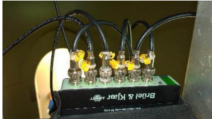
LAN-XI unit attached to the ladder
