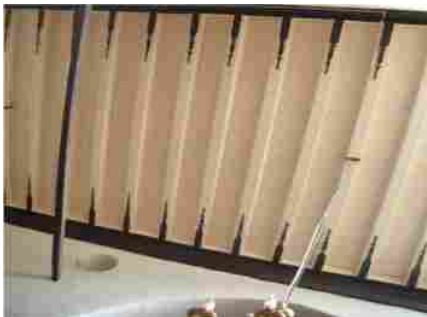
Pl. 24. The ceiling wooden braces, Hilal Mosque
