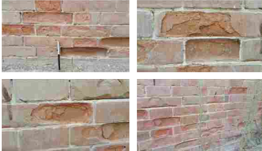
Figure 29: Shows the effect of soluble salts in conjunction with cement mortars and vegetation on the palace walls
