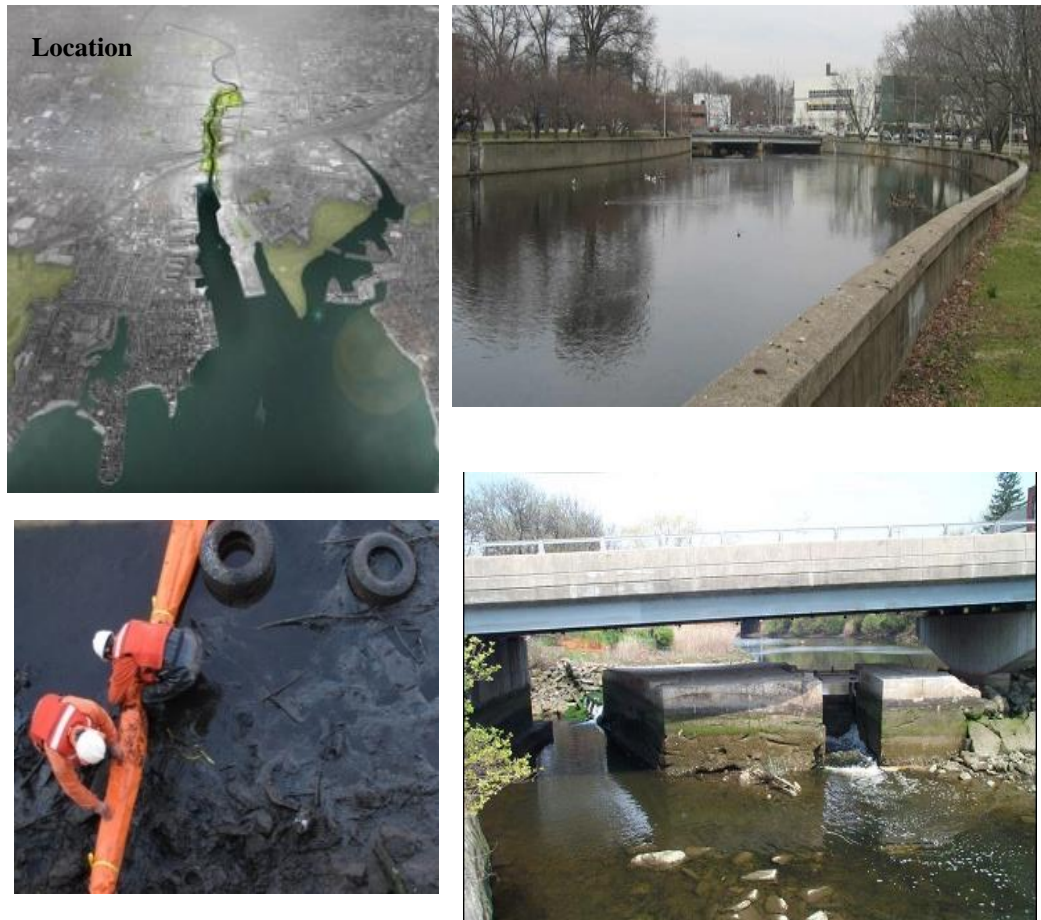
Figure (6) The Mill River condition prior to the project
