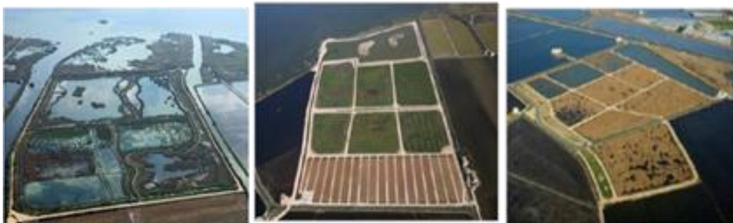
Figure (11) The 3 constructed wetlands of Albufera
