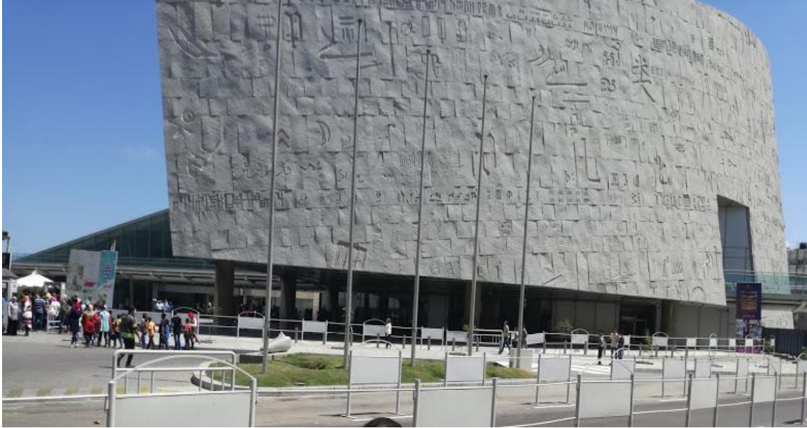
Figure (19) Three more Security Fences surrounding the Library Area
