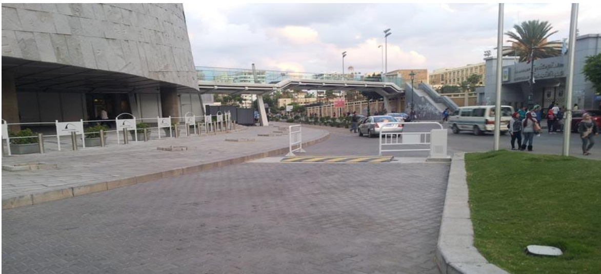
Figure (18) Increasing another Security Fence around BA area
