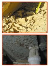
**Photo 5.** Effect of rain water at the ceiling and inside tombs at Bani Hassan.
