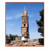
**Photo 2.** Effect of wind erosion at El Bahnasa site (Minaret Abu Samra).
