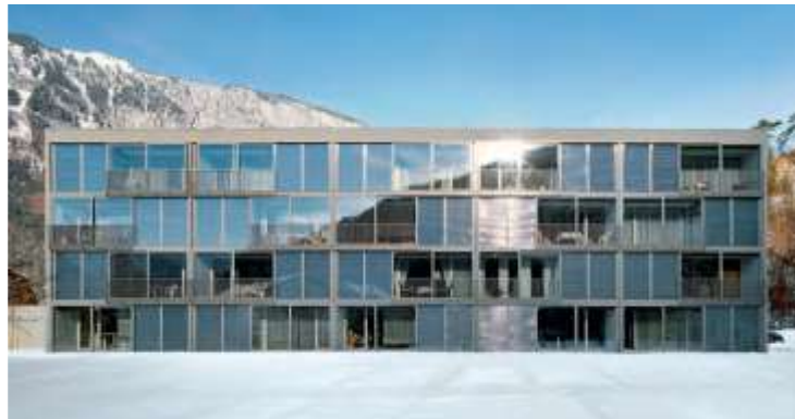
Figure (6) South façade of the apartment building- Switzerland [3]
