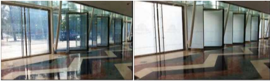
Figure (15) PDLC glass for the front elevation-East Wintergarden venue, London [11]
