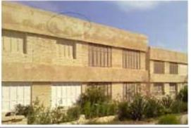
Moisture damage by rain and UV: High water absorption during driving rainfall months: parapets absorb most water, and dry out unevenly, leaving wet patches, and efflorescence, color bleach of wall render caused by long exposure to UV radiation externally
