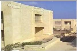
Moisture damage by rain: Efflorescence and wet marks
