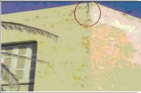
Heat Damage by solar radiation: Corner cracks in parapet walls due to thermal expansion in non-Cladded buildings. Loss of Pigmentation due to UV Radiation.
