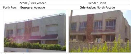
Moisture damage by rain: Limestone and brick cladded parts of the façade (including corners) were in a very good condition Moisture damage by rain:
