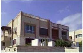
Moisture damage by rain and humidity: Cladded parts of the wall were found in a very good condition
