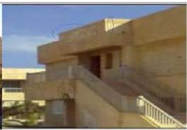
Moisture damage by rain and humidity: Efflorescence on parapet wall - and at ground floor walls exposed to garden's moisture and surface water. Step Crack at the corner of stair case side wall
