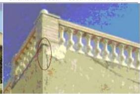
Heat Damage by solar radiation: Render finished Southern walls: Cracks at corners due to thermal expansion in noncladded buildings. Loss of Pigmentation due to UV Radiation.
