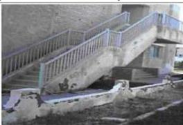
Moisture damage by rain and irrigation system: Faded color due to high exposure to UV. Slight cracking at the corner of parapet wall-severe damage to render layer (at the staircase side /parapet wall), at the parts where accumulated driving rain water over flow and fall off the wall side, causing complete wetting of the stair case walls
