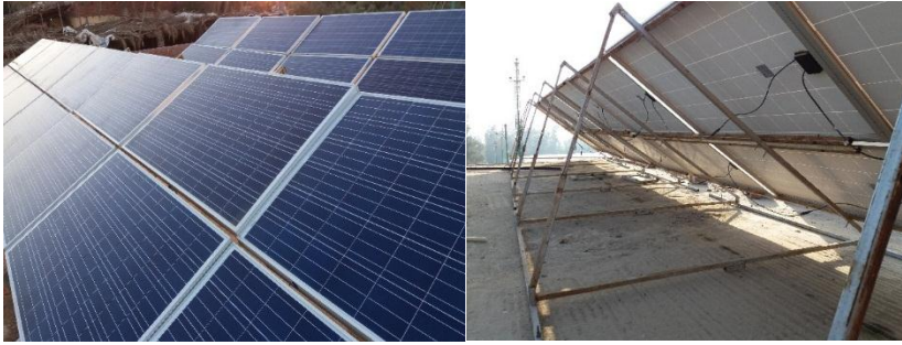
Fig. 1: The two sets of arrays and metal installation structure.
