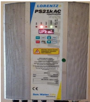
Fig. 2: The inverter.
