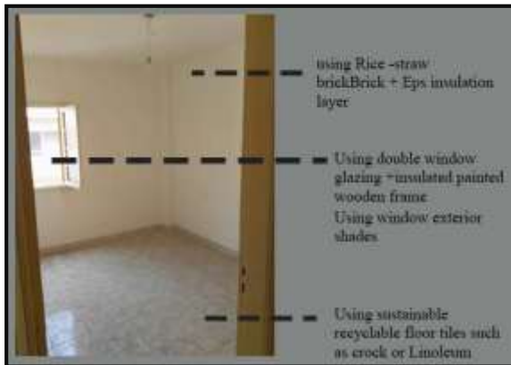
Fig. 30. The Proposed Modification of Building Material
