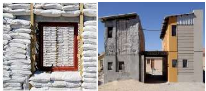
Fig. 12. Construction material of the Exterior wall
