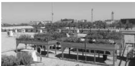
Fig. 3. Faculty housing's green roof. [16]
