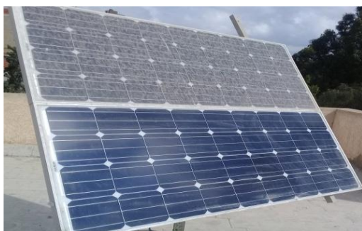
Fig (2) Clean and unclean for PV modules
