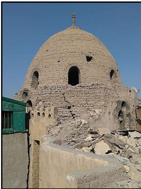
Pl.III The western façade
