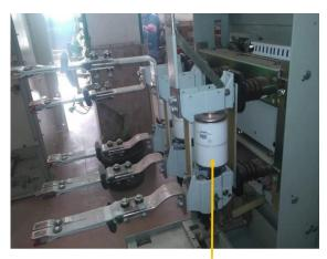
The expansion chamber **Fig.5.** The expansion chamber of circuit breaker
