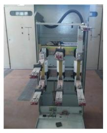
Fig.4. The circuit breaker (SF6).
