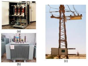
**Fig.3** Electrical distribution network components of interest: (a) Circuit breaker (b) Transformer (c) Automatic recloser.
