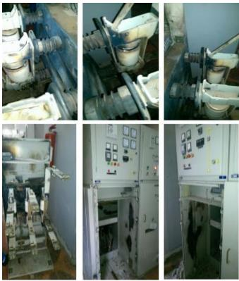
Fig.7. Explosion of the Expansion Chambers Effects
