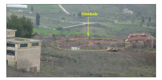
Figure 3: Sinkhole ISPEA mine
