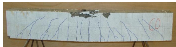
Fig. (8) Mode of failure of tested beam C0
