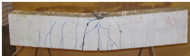
Fig. (4) Mode of failure of tested beam A0
