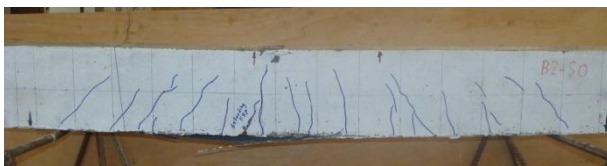
Fig. (4) Mode of failure of tested beam B2-S0
