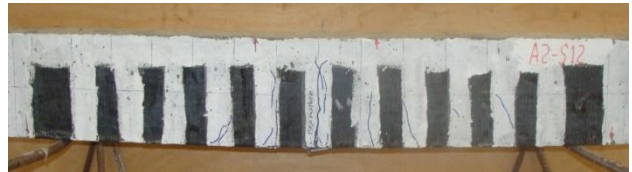
Fig. (7) Mode of failure of tested beam A2-S12
