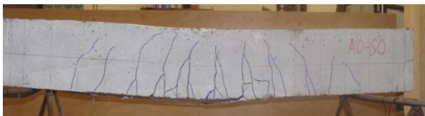
Fig. (3) Mode of failure of tested beam A0-S0
