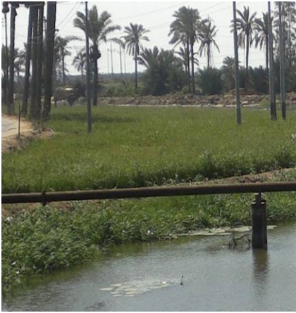
Fig. 7. Low level area of about 300 feddans upstream of gamasa weir, and embankment level is about (1.00) m
