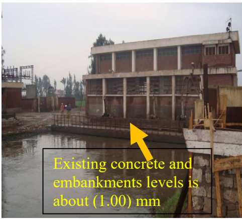
Fig. 8. The delivery basin of pump station No. 2
