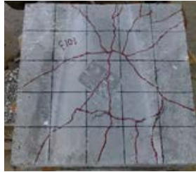
Fig. 19. Fracture mode of 10% FRAC under flexural load.
