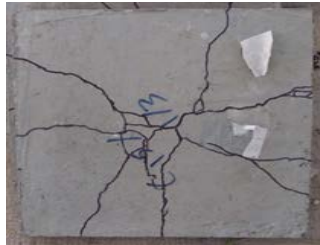
Fig. 26. Fracture mode of 15% CRAC under flexural load.
