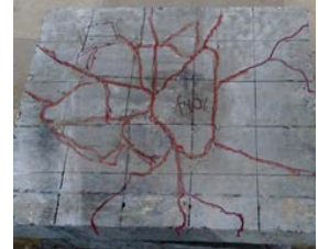
Fig. 24. Fracture mode of 40% FRAC under flexural load.
