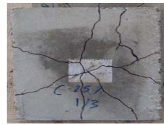
Fig. 27. Fracture mode of 25% CRAC under flexural load.
