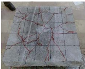
Fig. 23. Fracture mode of 30% FRAC under flexural load.
