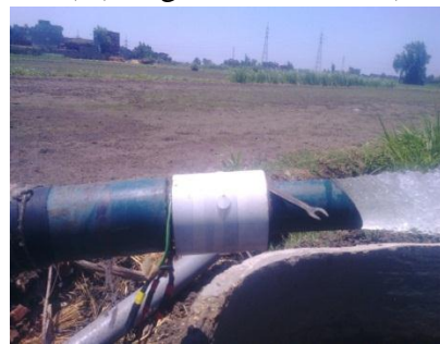
Fig.2: The electromagnetic outlet irrigation pipe.
