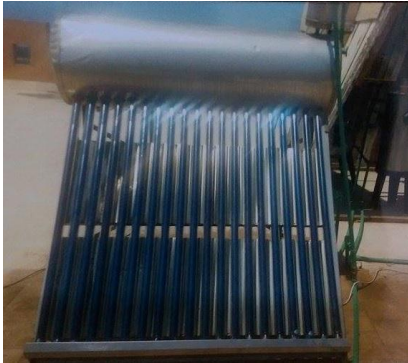
Fig. (1). Photo of evacuated tube header collector
